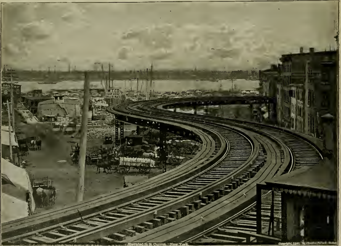
Fig. 6. A CROOKED PORTION OF THE ROAD, THIRD AVENUE "L."
